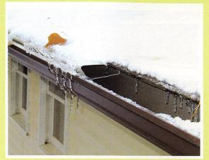
As pictured, ice and snow rests on <u>top</u> of *LEAFPROOF®*, but it will collect in an unprotected gutter. Eventually the ice and snow that has collected in a gutter will severely damage the gutter, soffit and fascia. The potential damage that will occur may greatly exceed the cost of the *LEAFPROOF®* installation.
